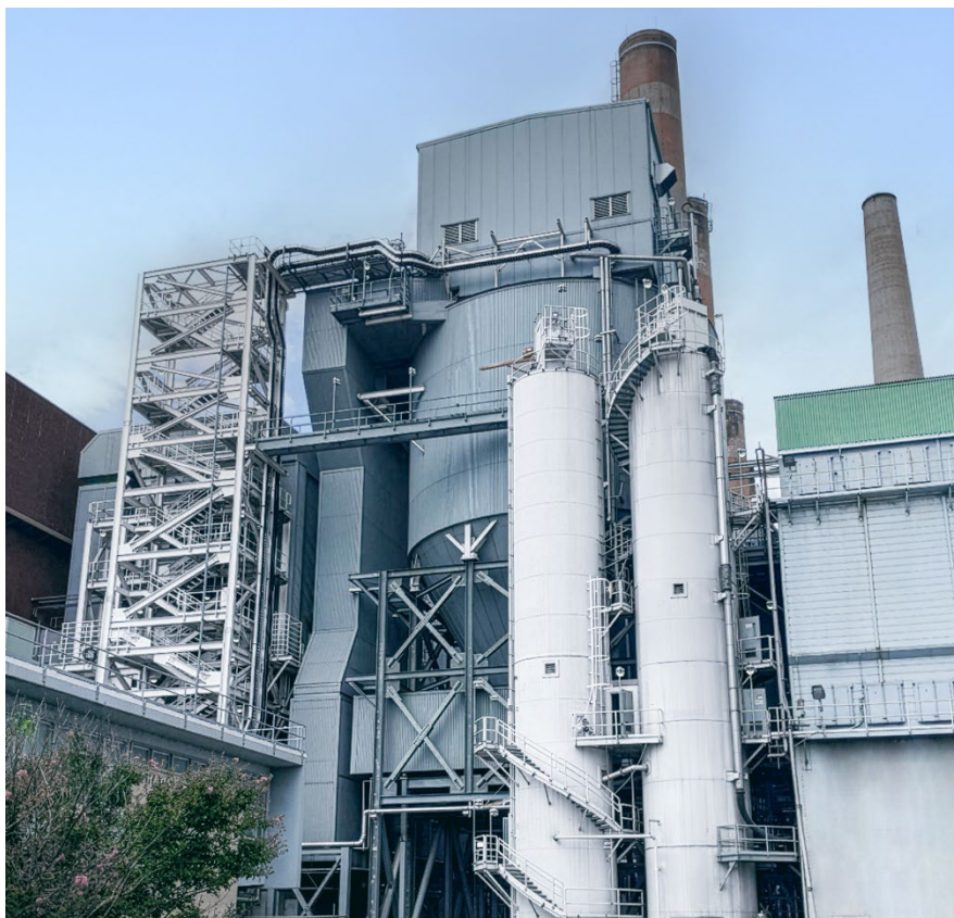
SDA System on TVA Shawnee Plant Boiler Unit 1
